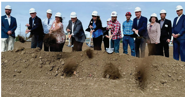
SUN PRAIRIE LOCATION GROUNDBREAKING
